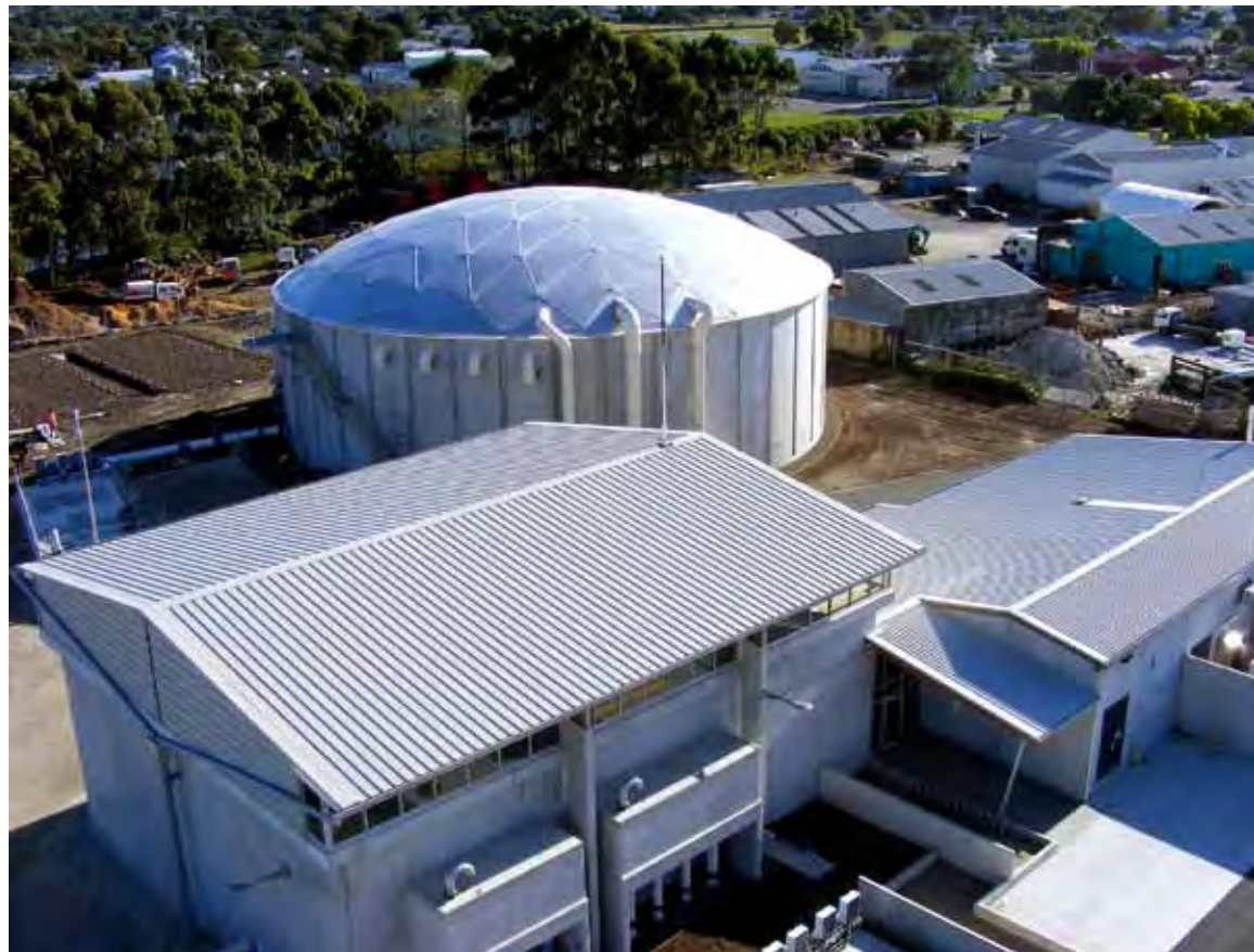
Elevated view of the WWTP on Banks Street.
